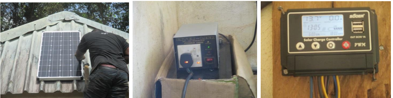
Solar Power for the Water System Too; An independent solar system was installed to run the UV-C light that purifies the water in the Aqua Pura Waterflow system.
